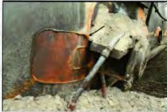
Photo 18. Damaged stub sill
