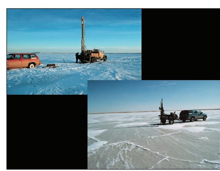
during the Winter in 1996. The drillholes ranged in depth from 10 to 54 feet. Sample collection via coring was troublesome due to the presence of lacustrine clays, noncohesive silts, and well indurated crystalline salt beds. Mobil B-50 HSA rig was used to initiate the drilling operation. After a mechanical failure, unrelated to the drilling activity, a trailer-mounted Giddings soil probe was used to complete the drilling operation.
