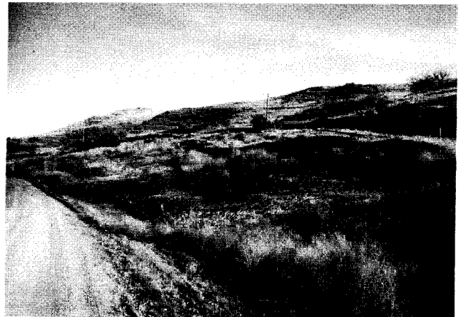
A slump or slope failure in Hell Creek strata (right of road) just north of Huff Hills Ski Area. Most slope failures in this area occur in bentonites (swelling clays) within the Hell Creek Formation.
