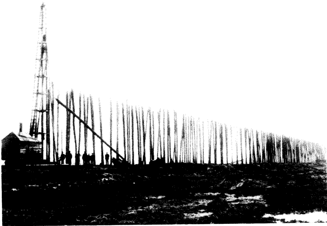
Figure 2. Driving piles for the Stockwood Fill (circa spring, 1906). S.P. Wange photo, Clay County Historical Society.
