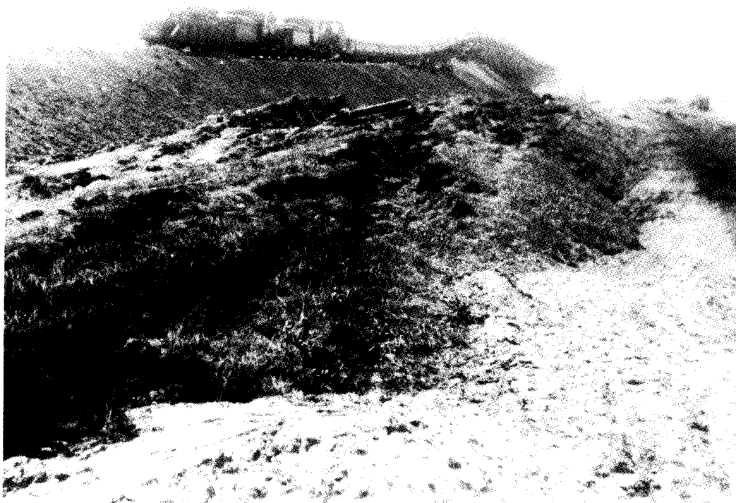
Figure 7. Filling trestle near concrete archway (circa June, 1909). View is to the southwest. A.F. Rusten photo, Clay County Historical Society.
