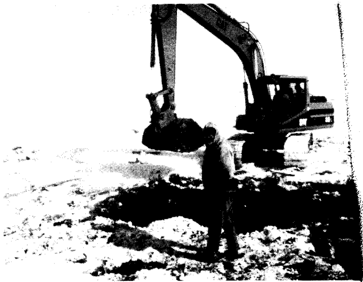
Figure 4. Backhoe used to dig trenches in both outlets. Roger Johnson is pictured observing trenches being dug in his pasture in the Tolna outlet. Shown in the background is the truck-mounted Giddings soil auger. Photo by Ed Murphy.
