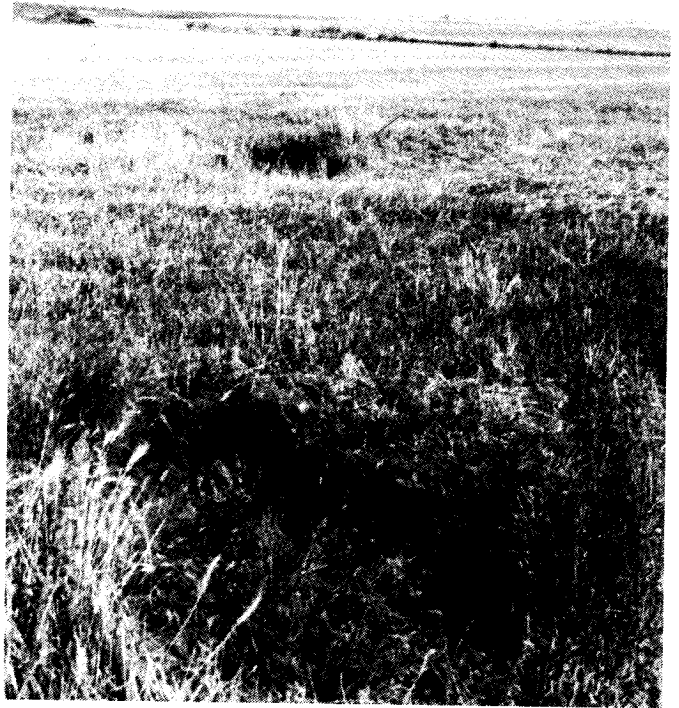
Two collapse features at the Keller Cave site. The holes are spaced 50 feet apart on a northwest-southeast trend. The holes may have an underground connection.
