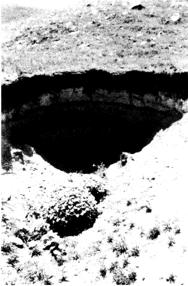
The collapse of a segment of an underground mine in the foreground has created a crawl space into a partially collapsed room at a mine near Haynes in Adams County.
