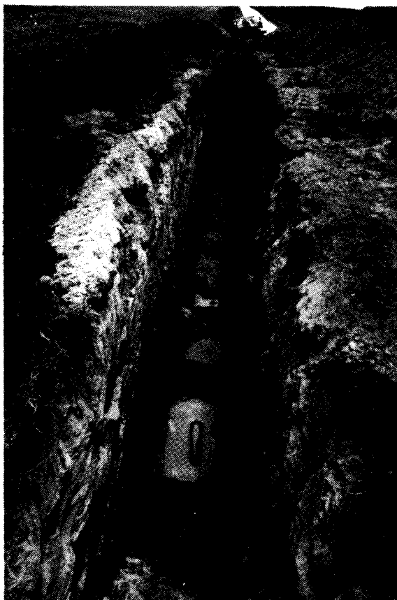
Figure 2. Backhoe excavation across Hogback Ridge. The trench was as deep as 15 feet and about 3 feet wide.
