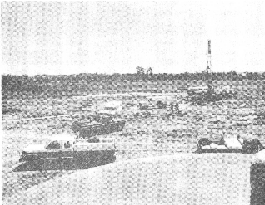
Installing monitoring wells in the brine pit study site in the Wylie Field, Bottineau County (1984).
