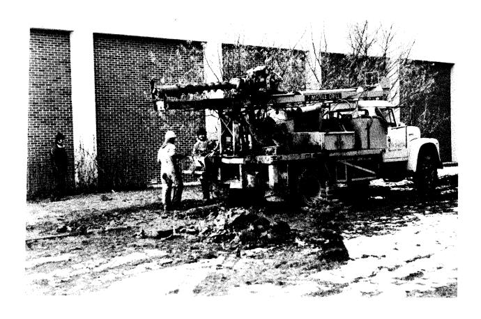
Mission accomplished! Our drill rig is a Mobile B-50, hollow-stem auger drill, capable of drilling depths of about 200 feet. A few equipment changes would allow us to rotary drill as deep as 1000 feet or diamond-core to 1400 feet. The rig has seen a great deal of use since we obtained it in 1975.
