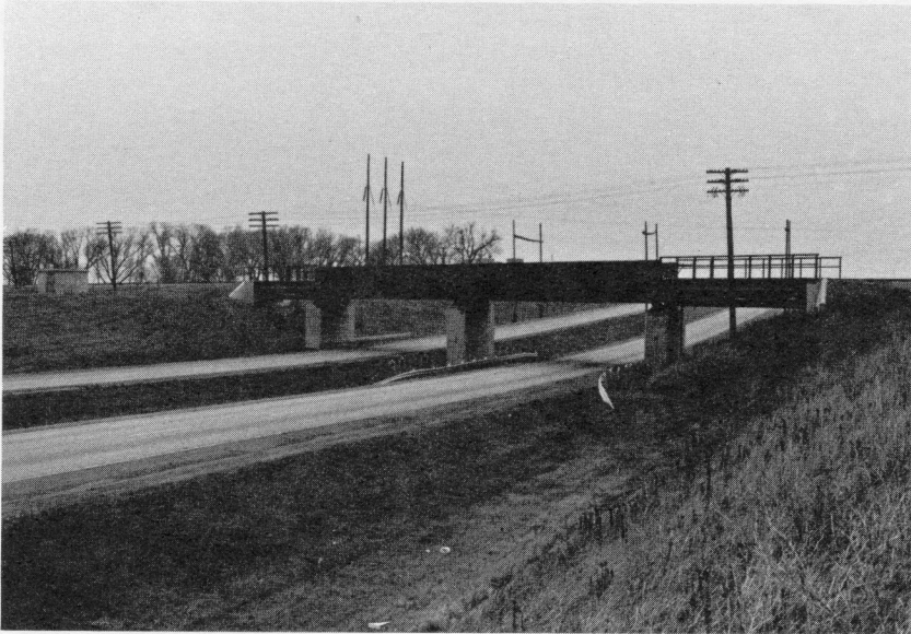
FIGURE 6. Construction of this railroad underpass was delayed because of failure to recognize a unique geologic situation.
