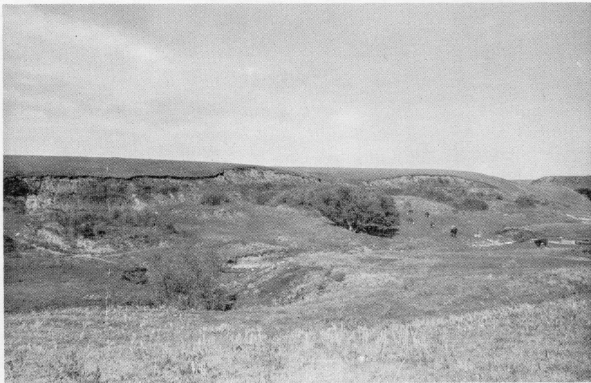
Figure 16 - Abandoned scraper operation now used as pastureland. Old spoil piles along bank (right center) are quite similar to slump blocks (center and left center) along bank. Location - Weigum Mine in SW SW of Section 20, T. 146 N., R. 89 W., Mercer County, North Dakota.
