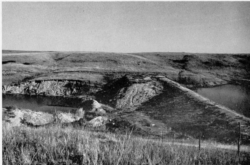
Figure 14 - An earth-fill dam using spoil pile material to provide a stock watering pond. Location - Ledahl Mine in NE of Section 10, T. 154 N., R. 100 W., Williams County, North Dakota.
