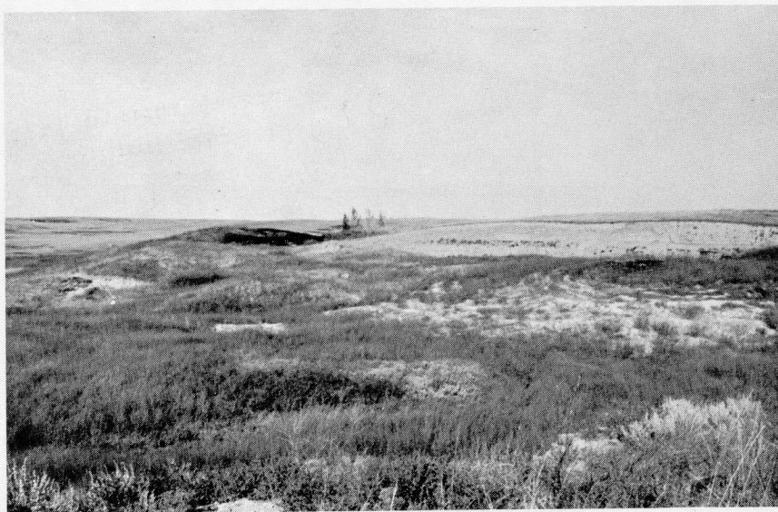
Figure 12 - View of recently active dozer and scraper operation. Pitwall in center background, spoil piles in center foreground are partially covered with vegetation. Location - Landaker Mine in SE of Section 21, T. 153 N., R. 90 W., Mountrail County, North Dakota.
