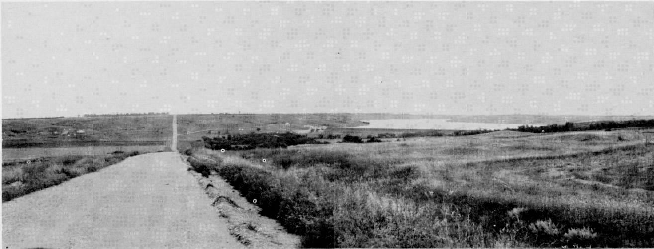
Fig. 1 - View of Bald Hill Dam and Lake Ashtabula from stop 2. Farm across valley sits on Pleistocene terrace of the Sheyenne River.
