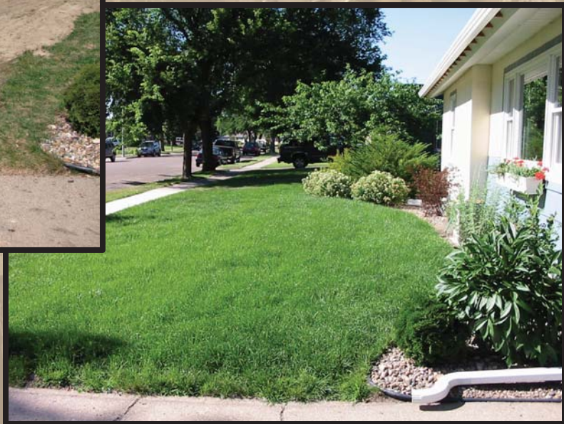
Figure 5 (right). Two-and-a-half months later. There is no surface indication of the well field at all. Some ground settling may occur over the winter but that is easily corrected. Externally, our geothermal system is, to all intents and purposes, completely invisible.
