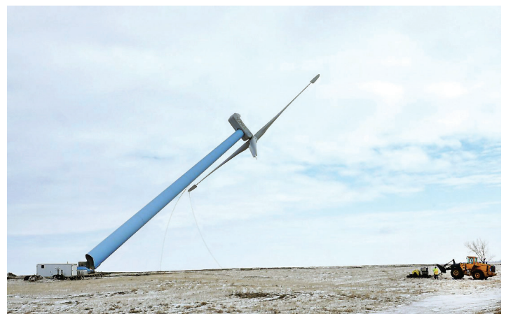
FIGURE 4. Decommissioning of the first wind towers in North Dakota south of Minot. This process is called chop and drop, similar to felling a large tree, where the base of the tower is cut and the tower is pulled over with cables and heavy equipment (Image by Jill Schramm, Minot Daily News).
