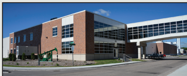
Figure 1b. Recently renovated core library in 2016. Steam plant and parking lot on the right may be compared to Photo 1a for reference.
