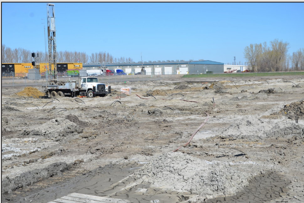
Figure 2. A shallow, closed-loop geothermal system being installed at the Minnkota Power Cooperative site in Grand Forks during the spring of 2016. A total of 646 wells were each drilled at this site to an approximate depth of 285 feet.
