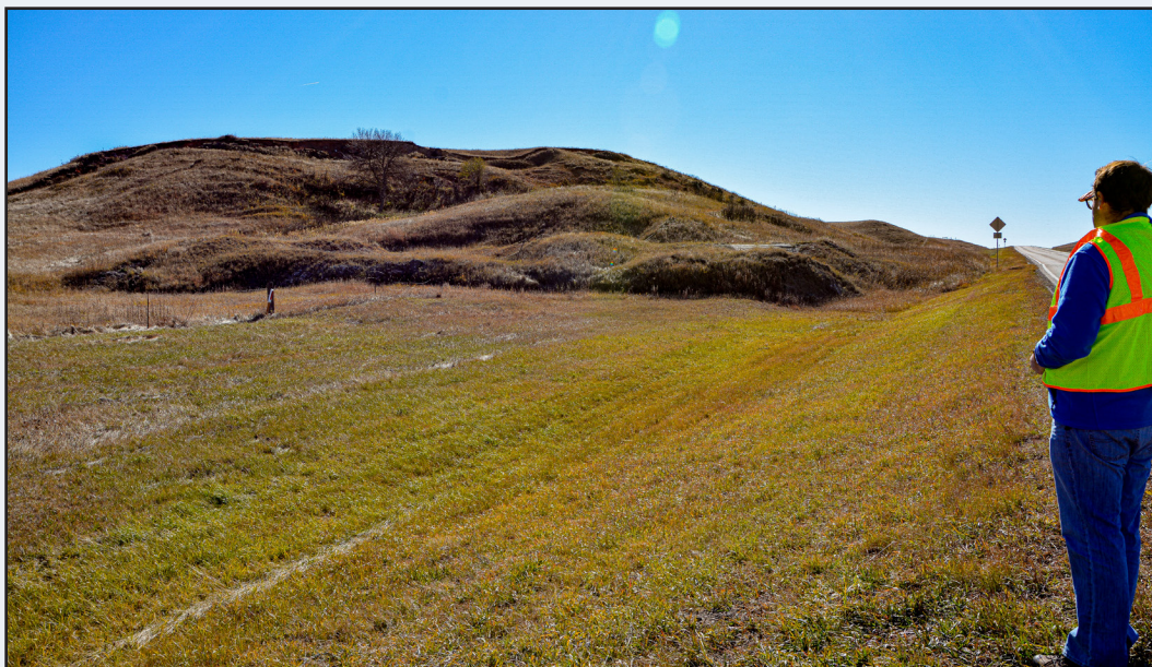
Figure 4. NDGS Geologist and FAA Part 107 Pilot, Chris Maike, examining a landslide impacting ND Highway 49.
