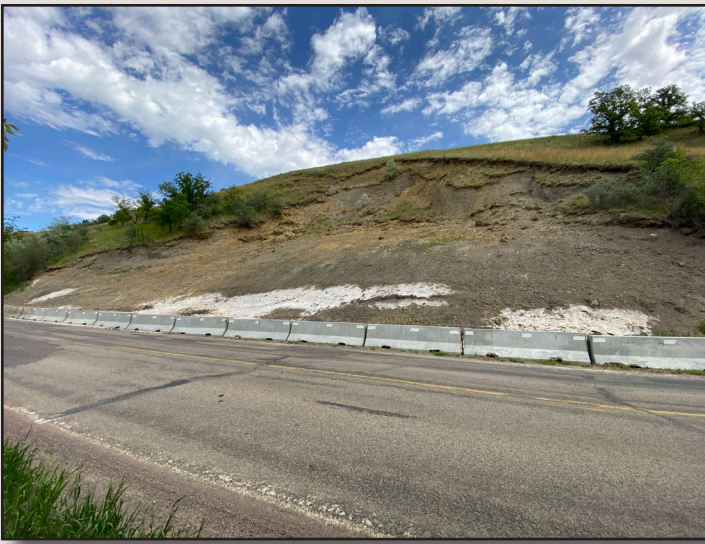
Figure 2. Groundwater seeping out of the base of the remediated hillslope along River Road in June of 2020. White-colored alkali minerals show where groundwater reaches the surface and evaporates. This flow was likely a significant factor in the collapse of the slope.
