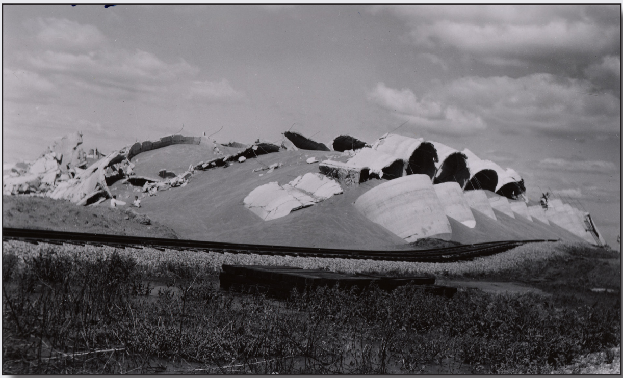
Figure 7. The Fargo Grain Terminal elevator collapsed around midnight on June 12, 1955, spilling 600,000 bushels of wheat and other grains. Image from the Institute for Regional Studies, North Dakota State University, Fargo, North Dakota.
