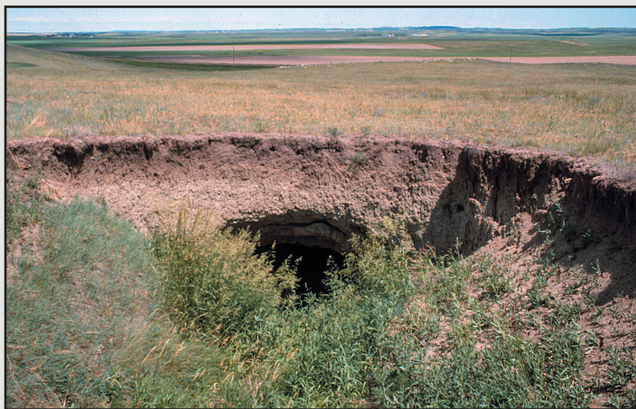
Figure 1. A five-foot-deep sinkhole caused by underground mining near Haynes in southern Adams County. The void visible along the back wall of the sinkhole represents the adjacent portion of the mine collapse working its way to the surface. The roof above it will soon collapse. NDGS photo by Ed Murphy in the 1980s, prior to reclamation of the site by the North Dakota Public Service Commission.
