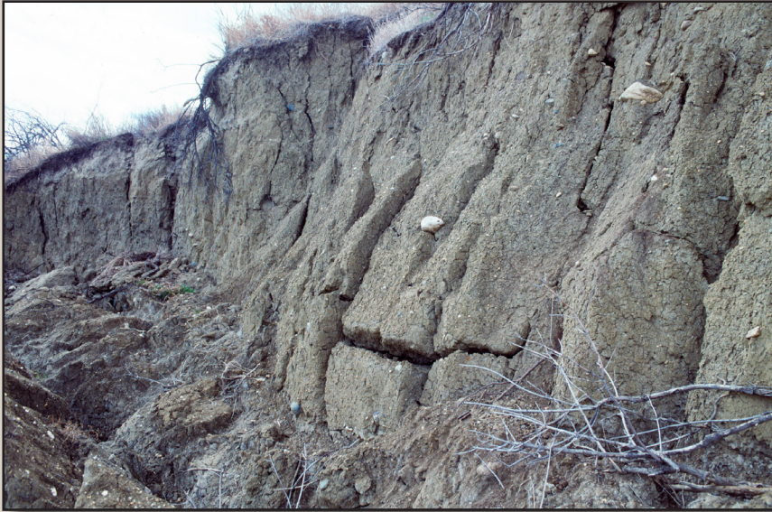
Figure 4. Jointed till in the scarp of a landslide north of the BNSF railroad tracks southwest of Williston. The slope below was littered with blocks of till that had toppled down the slope. I was investigating this slope in 1996 when the vibrations from a passing freight train caused a 6 x 8 foot block of till to topple from the scarp in the background.
