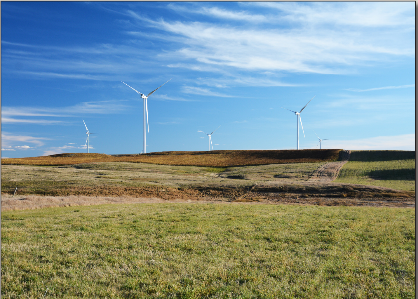
Figure 9. Newly installed wind turbines situated on a plateau in western Morton County.
