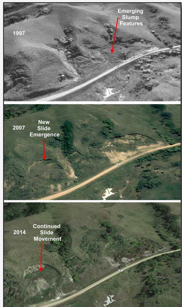
Figure 6. Pseudo-oblique images rendered in Google Earth of landslide features along County Road 80 just west of Huff, ND show the emergence and continued movement of these slides over an 18-year time period from 1997 to 2014. Employing a drone to periodically monitor areas like these along transportation corridors across the state could provide additional cost savings by detecting changes along engineered slopes prior to large scale failure.
