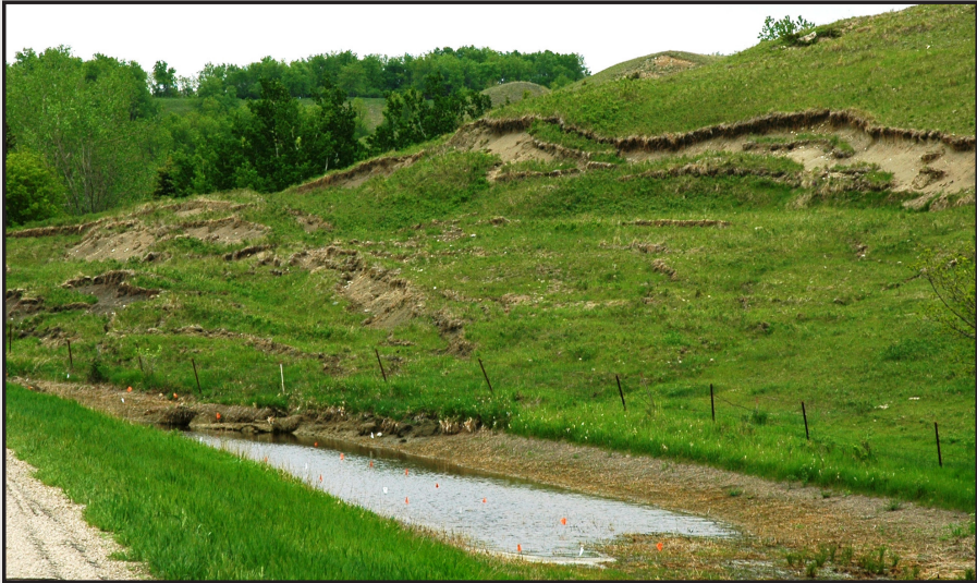
Figure 4. Landslide near Highway 21 south of Valley City in the Sheyenne River Valley. This slide damaged the fiber-optic line running in the ditch alongside the roadway.
