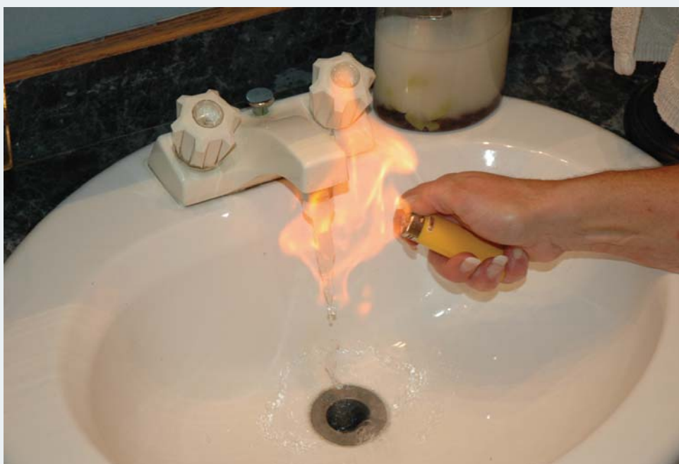
Figure 2. An ignitable natural gas show at the bathroom sink, produced by water from a well at the Mayer farm in northwestern McHenry County. Mrs. Mayer commented that her well has produced groundwater with ignitable quantities of natural gas for several decades.
