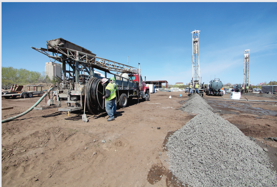
Figure 1. Three truck-mounted drill rigs were used to construct the well field for the 100,000-square-foot addition to the Heritage Center. The truck in the foreground has its drill mast lowered while the crew maneuvers a loop reel into place. The reel holds a ground loop assembly, consisting of a prefabricated U-bend fused to two lengths of HDPE piping. After it is inserted into the borehole, the loop will be grouted in-place with a specially formulated thermally-enhanced grout. Later on, the individual ground loops will be connected into five separate closed circuits via headers buried about 6 feet below the ground surface (see figs. 4-7). Each circuit will have its own supply and return lines to and from the interior part of the geothermal system. The gray mounds to the right of the truck are drill cuttings piles. (Photo by Brian Austin, SHSND)
