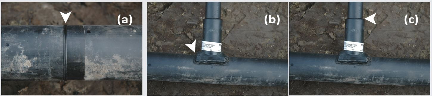
Figure 5. In the field, all plastic pipe joints are thermally fused. Originally developed for connecting HDPE gas lines, heat fusion is a process in which two melted pipe surfaces are brought together and held in-place under gentle pressure until resolidification is complete. As it cools, the molten plastic from each surface fuses into a homogeneous mass, effectively creating a seamless joint whose thicker walls make it not only stronger than the rest of the pipe, but virtually leak-free as well. Two methods of heat fusion commonly used for headering up are butt fusion and socket fusion. Butt fusion is a form of plastic welding: the technology responsible for much of that seemingly ubiquitous and infuriatingly hard-to-open plastic packaging we all know so well. Butt-fused joints are formed between two pipe ends and are commonly used on main header lines (a). A variation of this procedure called saddle (or sidewall) fusion is used to join concave and convex surfaces, such as an adapter fitting to the side of a pipe (b). Most header pipes arrive from the manufacturer with the saddle fusion joints already in-place. Socket fusion is used to connect small-diameter pipe (ground loops, for example) to socket fittings (c).
