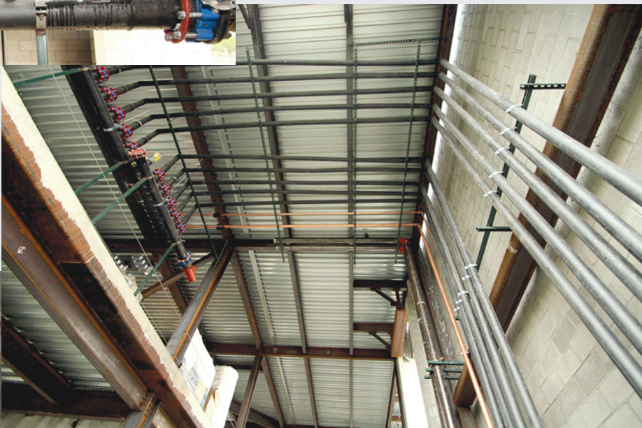
Figure 2. Header arrangement inside the building. This is where the supply and return lines to and from the well field come together. Although it is difficult to see in this picture, there are two separate headers (the large horizontal pipes) – one for supply, the other for return. Each pair of lines is connected to the headers by shut-off valves (the blue-and-red objects) that will allow isolation of the individual well field circuits for finer control of the building's climate and for maintenance. (Photo by Brian Austin, SHSND)
