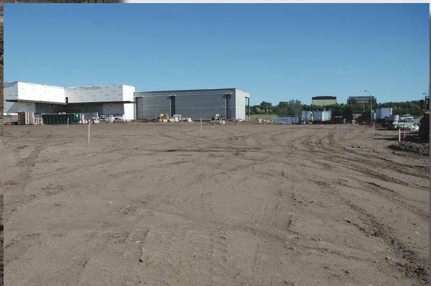
↓ Figure 7. The completed well field, smoothed and leveled, against a backdrop of the Heritage Center addition's main entrance (behind the dumpster) and Governors Gallery (right). The surface will eventually be paved and made into a parking lot and loading area.
