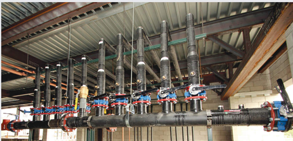
Figure 3. The same headers viewed from below. The supply and return lines for the well field are clearly visible where they cross the ceiling and extend down the wall on the right. They run the full height of the building and exit through the ground-level floor. This rather lengthy up-and-over pathway is a consequence of the building's interior layout. It is not a requisite of the GSHP system. (Photo by Brian Austin, SHSND)
