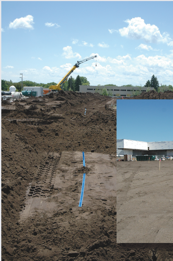
← Figure 6. Backfilling a header trench. Bright blue detectable warning tape installed 18 inches below grade marks the location of the buried pipe.
