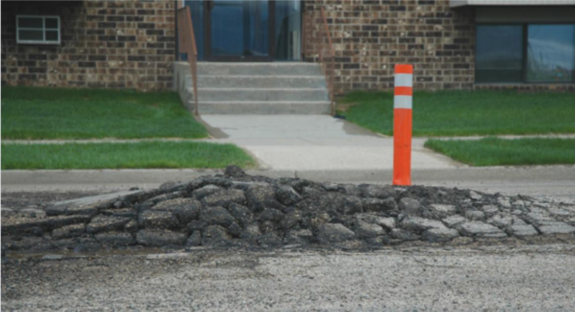
**Figure 3.** Spring 2011. Frost heave on this Bismarck street has lifted parts of the road surface about 18 inches (46 cm). The maximum freeze depth in the Bismarck area for the winter of 2010-2011 was about 40 inches (100 cm)\* (North Dakota State Climate Office, 2011). Photo by Lorraine Manz.
