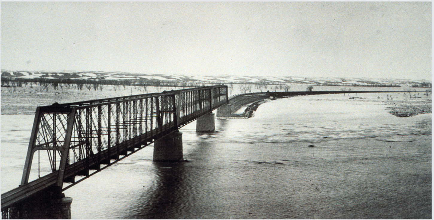
Figure 5. The Missouri River flooding in the spring of 1884. Water extends all the way from the railroad bridge west to the present location of ND Highway 1806 south of Mandan. The ice breakers on the middle piers are under water indicating that the water level exceeded 1,644.4 feet. These original bridge spans were replaced in 1905 because they could no longer safely support the ever-increasing weight of locomotives. Photo courtesy of the State Historical Society of North Dakota.
