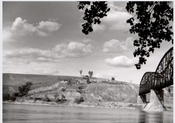
Figure 6. Several landslide scarps are visible along the east slopes of the Missouri River Valley above the Bismarck Railroad Bridge. The top of a City of Bismarck water reservoir is visible just below the largest tree at the top of the east slope. Photograph taken by Ralph Peck in 1951.
