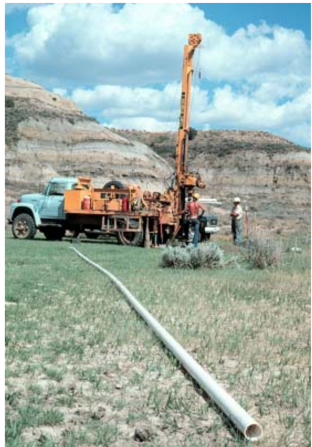
A 40-foot monitoring well is assembled and ready to be snaked down a borehole on a reclaimed oil and gas pad in western North Dakota in this 1980 photograph.
