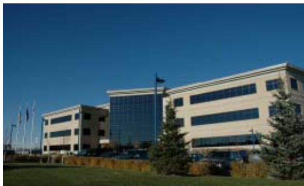
Figure 7. The Century Center in Bismarck is the largest state building in North Dakota to have a geothermal heating and cooling system.
