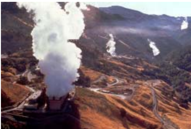
Figure 2. The Geysers Geothermal Field near Santa Rosa, CA obtains its heat (at about 330° F) from a large magma chamber about 4.5 miles below the earth’s surface. It is the largest producing geothermal field in the world, producing enough electricity to meet the demands of a city the size of San Francisco. (Photo courtesy of Pacific Gas & Electric and DOE/NREL).
