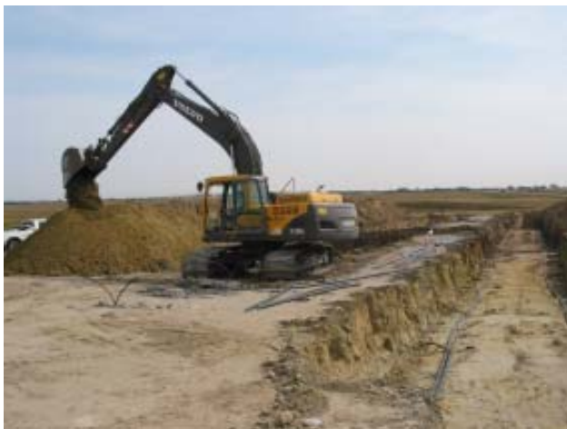
Figure 5. After the wells are completed, a trench is dug to a depth below the frost line and the well heads are connected to a horizontal "header" pipe that carries the heat transfer fluid to and from the heat pump. Depending on the number of wells, more than one circulatory zone may be constructed, enabling operation only of as much of the well field as is required to maintain the building's temperature at the desired level. (Photo by Tom Torstenson)
