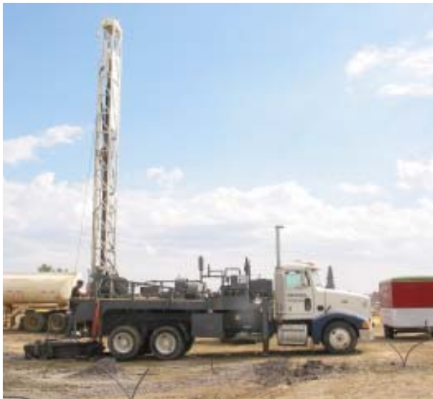
Figure 4. A truck-mounted drill rig is used for the construction of the wells in a vertical geothermal loop field. The V-shapes in the foreground are tops of the pairs of HDPE piping (the loops) protruding from finished wells. (Photo by Tom Torstenson)
