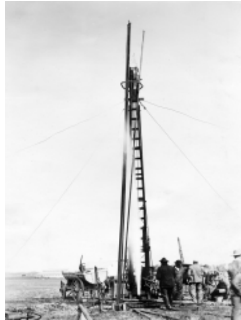
Fig. 1. Gas flowing from a well in north central North Dakota during the 1920's
