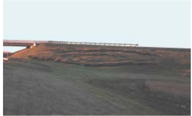
Figure 1. Failure of engineered fill soils on the eastern ramp of the Business Hwy 94 overpass just west of the City of West Fargo. Failure occurred after recent heavy rainfall in the area during the fall of 2004 (Photo by Anderson).
