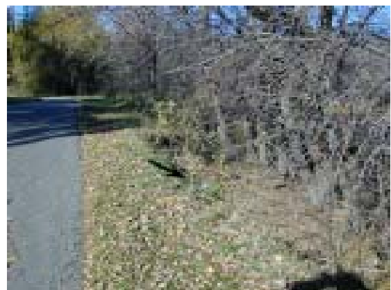
Figure 5. View to the north of failed cutbank along a meander of the Red River in north Fargo. Note the presence of a well defined failure scarp and the subvertical orientation of nearby trees (Photo by Anderson).
