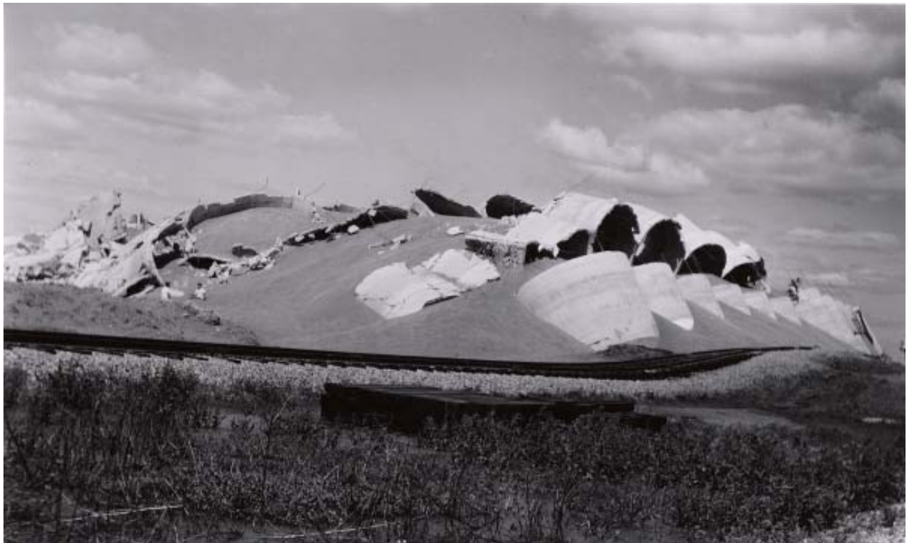
Figure 3. View of the collapsed Fargo Grain Elevator after subsurface soil failure in 1955. (Photo from the Institute for Regional Studies, NDSU, Fargo).
