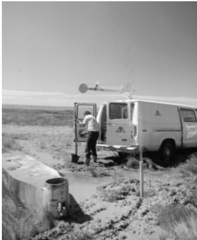
Figure 3. Gas blows from a newly installed monitoring well near the town of Lignite in northwestern North Dakota. The 2-inch well, drilled in 1984, was screened in a three-foot lignite at a depth of 90 feet. Gas did not start blowing until we had bailed about half of the mud out of the well. The gas blew for three days before it dissipated to the point that we could place a temporary cap on the well. The methane content of the gas was not determined.
