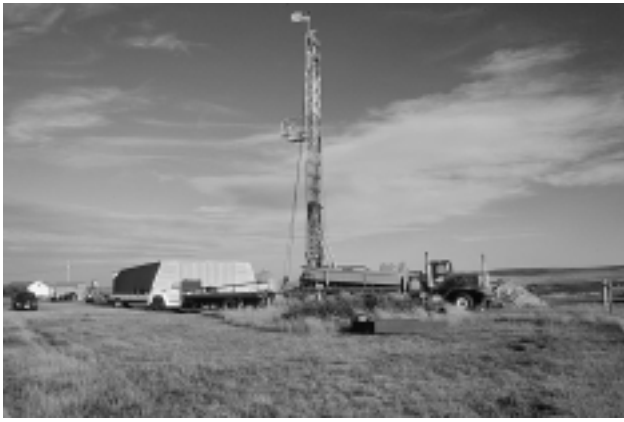
Figure 2. A truck-mounted rotary rig drilling for coal in western North Dakota.
