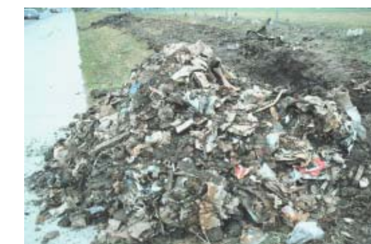
Municipal garbage, more than 30 years old, unearthed while installing buried cable along Century Avenue in 1998.
