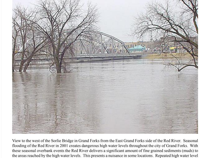
serve to weaken the bearing capacity of near-surface geologic materials (Photo by Bluemle).
