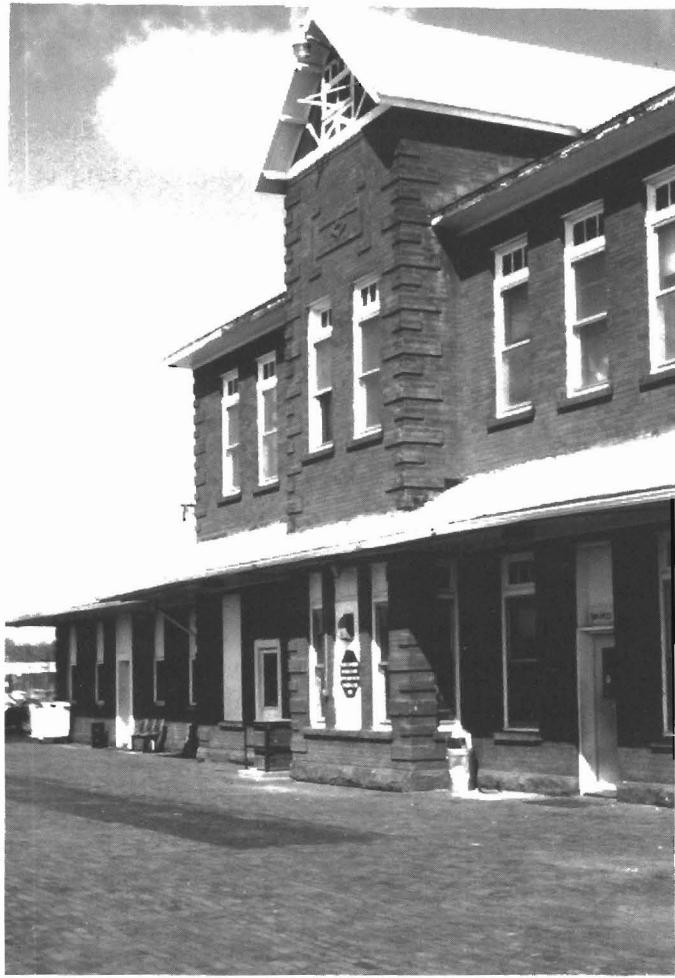
Figure 40. The Dickinson train station on Villard Avenue. The building was constructed from dark red brick that rests on a base of red sandstone blocks; window sills are also trimmed with this red sandstone. Crossbedded strata are readily visible in these partly hand-hewn blocks.
