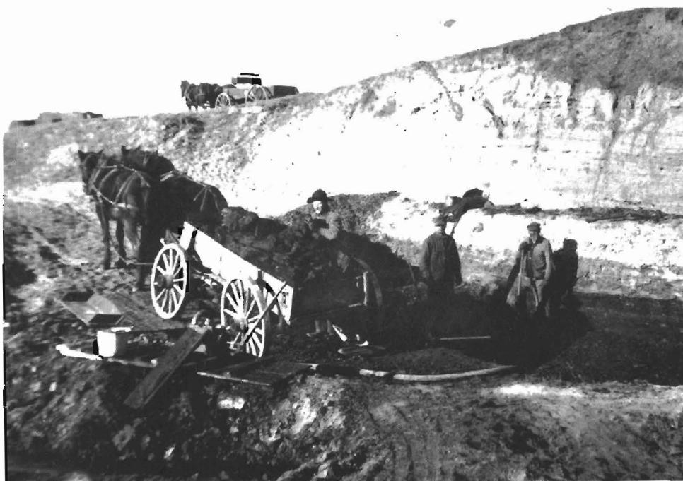
Figure 44. An early lignite mine along Spring Creek in southwestern North Dakota. These mines were generally referred to as wagon mines because farmers and ranchers would bring their own wagons to the mine to be loaded with coal. Photo courtesy of the North Dakota State Historical Society.
