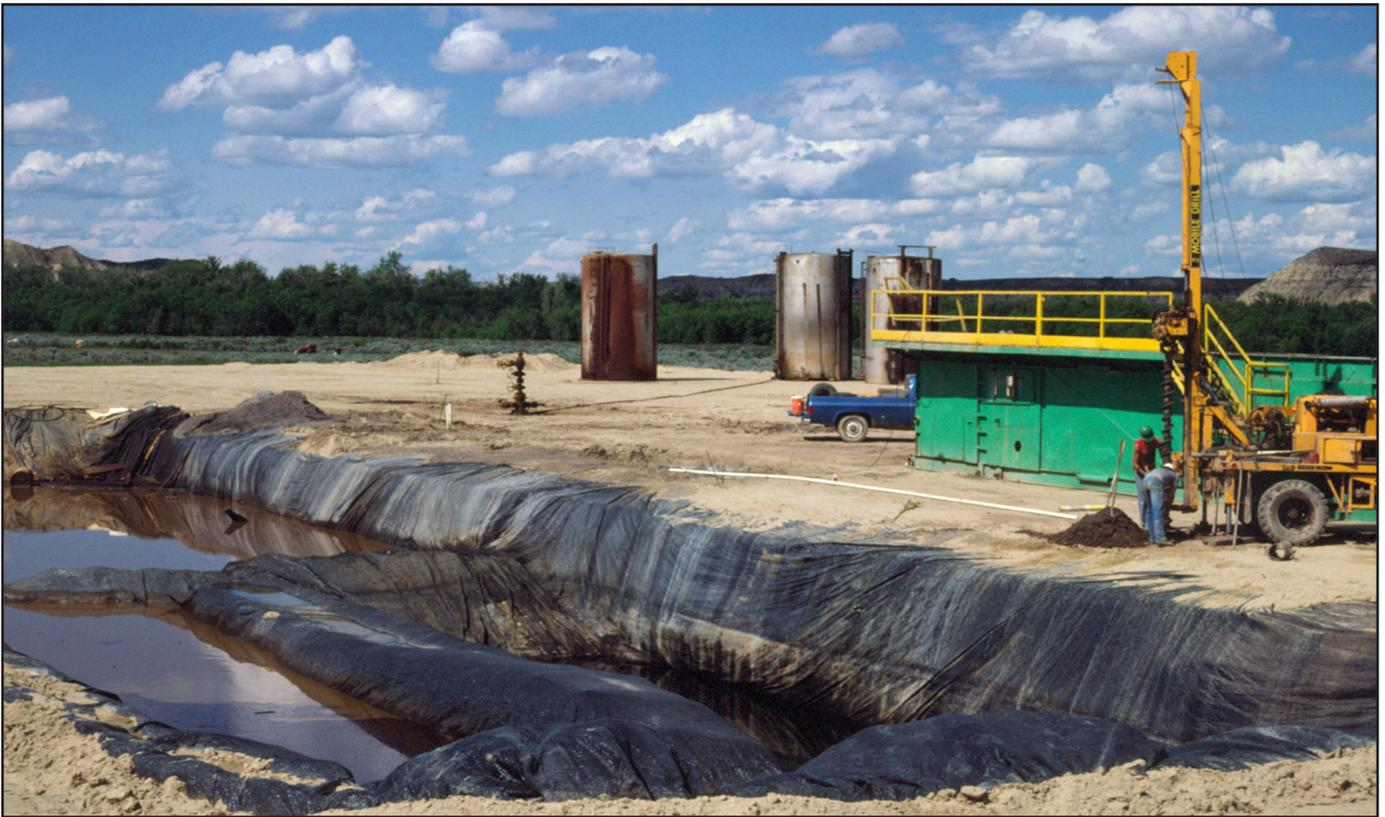
**Figure 7.** Monitoring wells in close proximity to buried drilling fluid. Above: Survey summer employees installing monitoring well no. 2 in 1981. Previously installed monitoring wells 3a and 3b are visible in the background. Below: Heavy equipment levels the reserve pit pushing drilling mud into the trenches. Wells 3a and 3b in the foreground.
