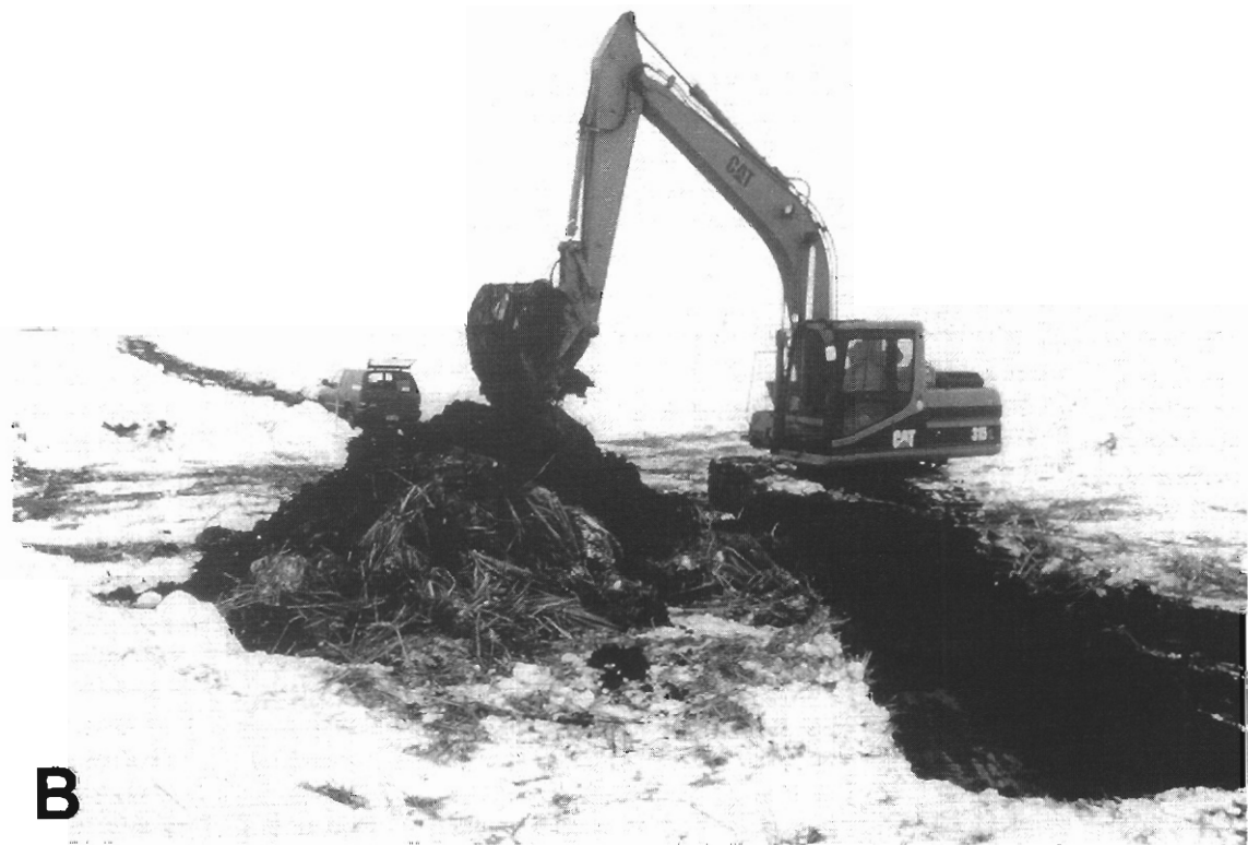
Figure 3. The truck-mounted soil probe (a) and backhoe (b) used to obtain sediment samples during this project. The photo of the truck was taken looking east from the Tolna site. The photo of the backhoe was taken looking southwest at the Jerusalem site.
