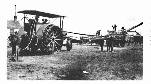
Figure 20. Threshing scene in 1919, near Mohall, North Dakota. A 60 hp. gasoline engine is pulling a 42" separator, the engine being operated by natural gas from the wellhead at the left.
