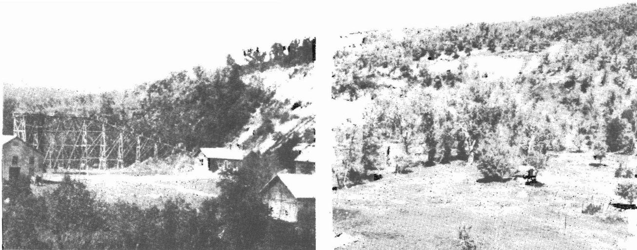
**Figure 15.** The Pembina Portland Cement Company plant at Concrete, North Dakota. Photo circa 1902-1909 courtesy of the State Historical Society of North Dakota (l). Recent photo of the abandoned site (r). The base of the kilns, building foundations, and scattered equipment are the only remains of the plant.
