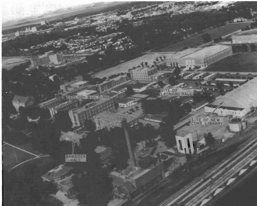
Figure 17. Air view of campus area in 1962 showing the geology building, Babcock Hall and sites of Leonard Hall and the new core library. The geology building housed the Survey and the Geology Department from 1948 until the expansion of the Survey staff following the discovery of oil in 1951. The Department then moved to Babcock Hall and the Survey was housed in the geology building until its move to Leonard Hall in 1964. Chester Fritz Archives.
