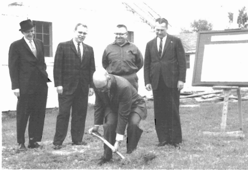
Figure 18. Dr. Wilson M. Laird turns the first shovel of earth for the construction of Leonard Hall on the campus of the University of North Dakota on September 16, 1963. Left to right, Myron Denbrook, architect, F. D. Holland, chairman of faculty building committee, Sulho Norri, Superintendent Lenci & Englund, Dr. George W. Starcher, President of UND.
