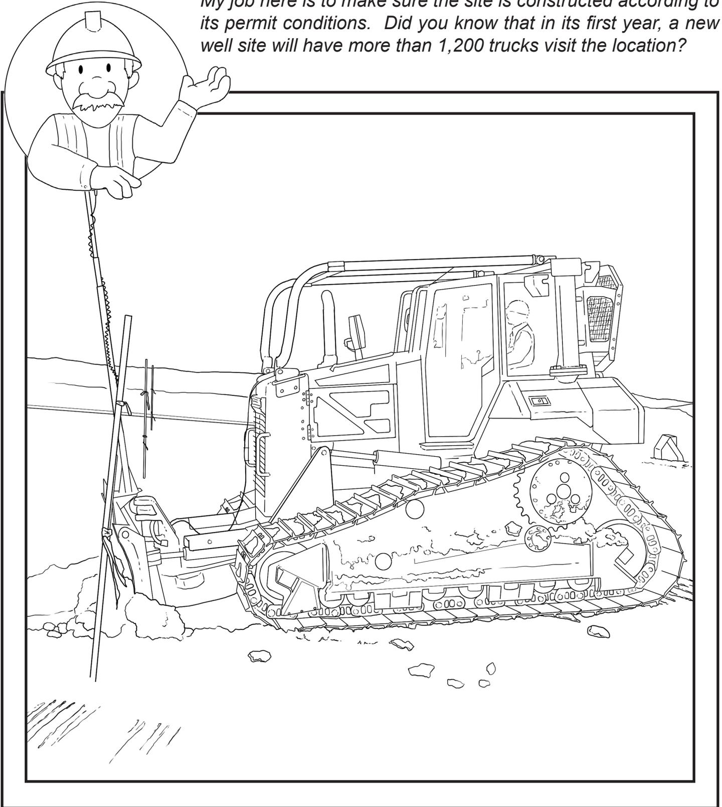
Here we are at a new location or drilling pad as it is being built. A small bulldozer works in between stakes which mark the spot where oil wells will be drilled. The work crew will level and compact the location then they will cover it with an orange rock commonly called scoria (though my geologist tells me it is not really scoria but a baked clay rock called clinker).
