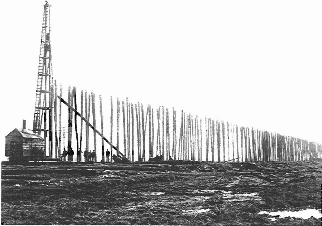
**Figure 2.** Driving piles for the Stockwood Fill, ca. spring, 1906. (S.P. Wange photo, Clay County Historical Society).
