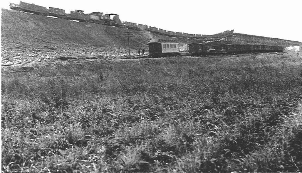
**Figure 5.** Attempting to fill the Stockwood Fill sink, ca. fall, 1907. View is to the southwest. Note the concrete archway ( $\approx$  at station #1262) at the right and the settling embankment at the left, forcing the tracks and trestle downward. (S.P. Wange photo, Clay County Historical Society).
