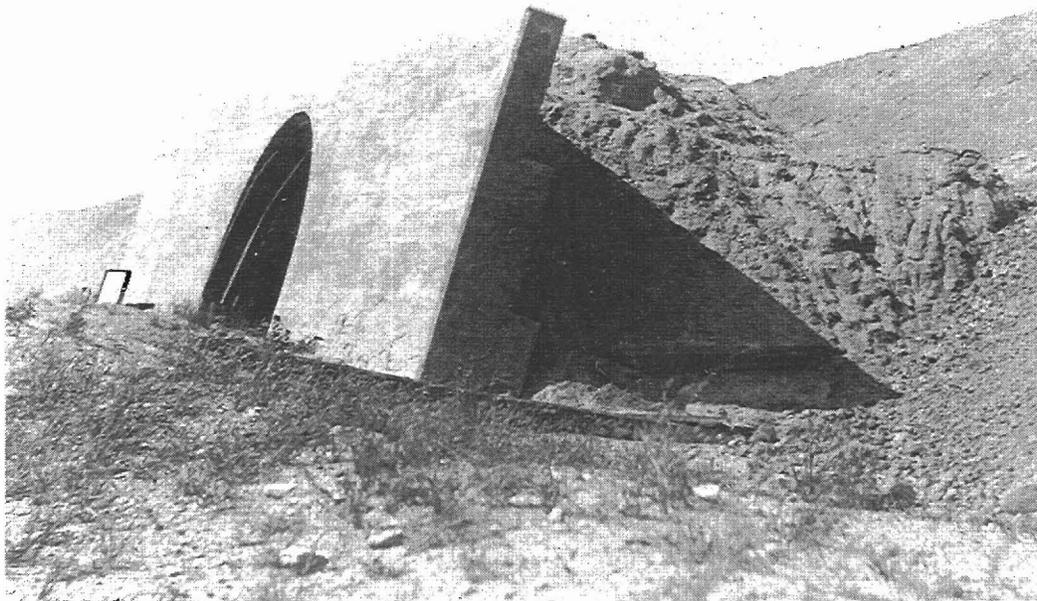
**Figure 8.** Collapsed archway, Stockwood Fill, ca. fall, 1909. View is to the northwest. (A.F. Rusten photo, Clay County Historical Society).
