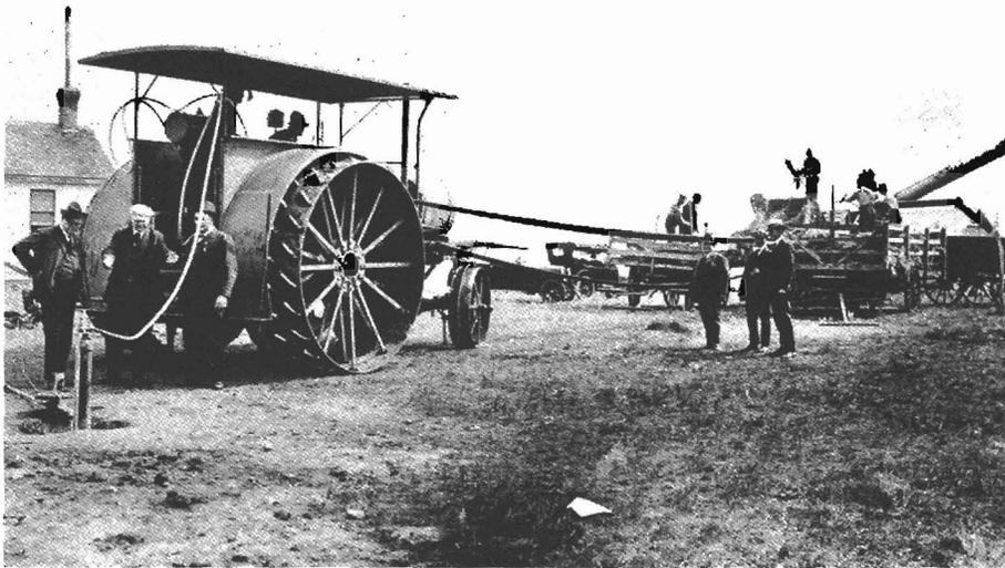
Figure 20. Threshing scene in 1919, near Mohall, North Dakota. A 60 hp. gasoline engine is pulling a 42" separator, the engine being operated by natural gas from the wellhead at the left.
