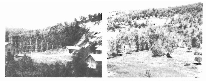
Figure 15. The Pembina Portland Cement Company plant at Concrete, North Dakota. Photo circa 1902-1909 courtesy of the State Historical Society of North Dakota (l). Recent photo of the abandoned site (r). The base of the kilns, building foundations, and scattered equipment are the only remains of the plant.
