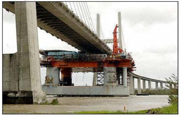
The PSS Chemul, a 13,000-ton semi-submersible accommodation/ maintenance vessel owned by PEMEX that broke loose during Hurricane Katrina is wedged under the Cochrane Bridge in Mobile, Alabama. (AFP/Stan Honda)
