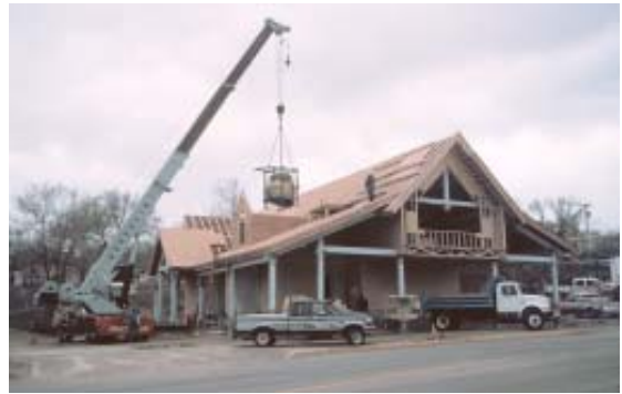
Lifting petrified tree stump through roof of Long X Trading Post.
