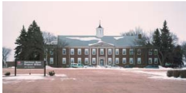
Figure 20. The U.S. Army Corps of Engineers Headquarters, Riverdale.
