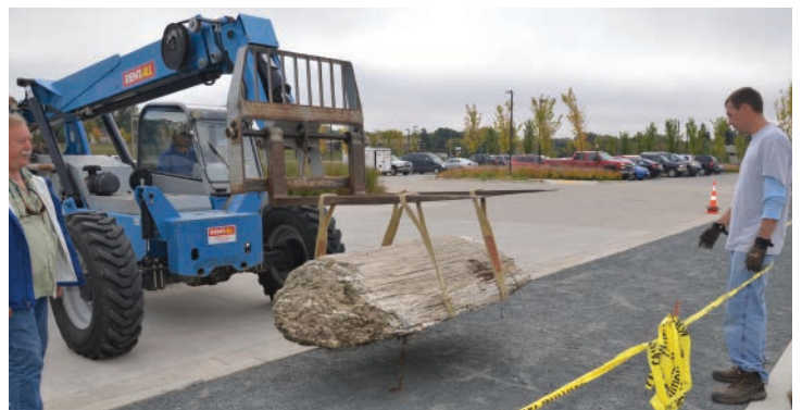
Tree and stumps moved with the cooperation of Straightway Construction.
