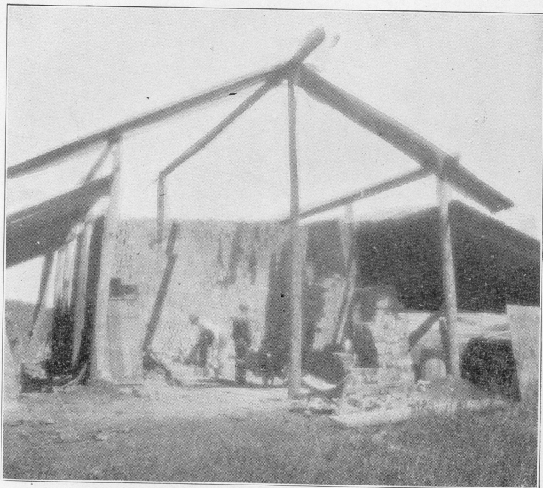
Scove kiln with permanent side walls, at Wilton Brick Plant.
