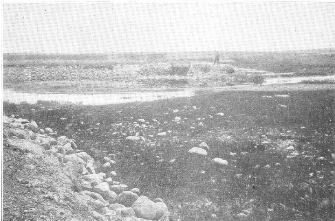
The Rounsaville dam on the Little Muddy above Williston
