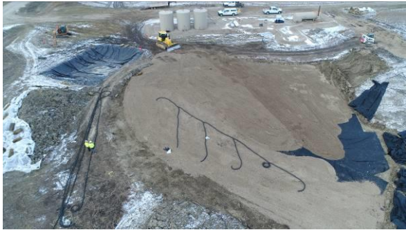
Photo #7 Installation of PVC drain tile in the capillary break with filter fabric.
