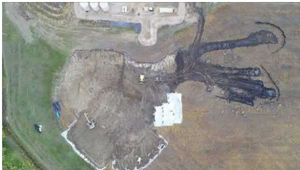
Photo #3 Stockpiling topsoil and excavated contaminated soil.
