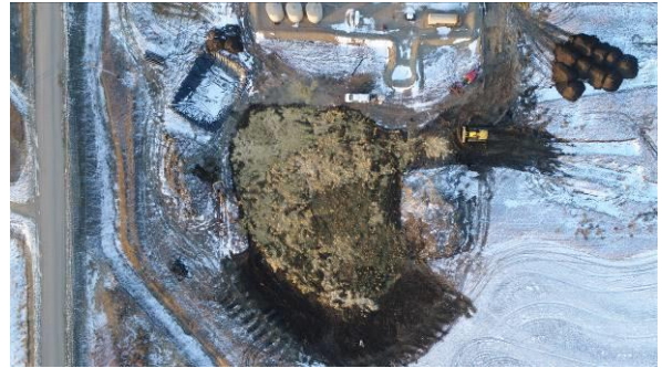
Photo #8 Placing gypsum and straw amended soil over capillary break.
