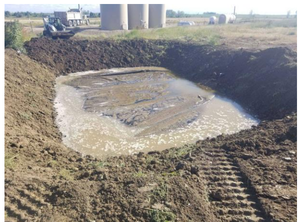
Photo #12 Placing soil cover over the Phytoremediation pond.
